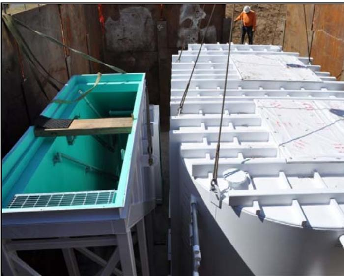
View from above as the stairwell and buried Flow Control Facility are being installed on a concrete foundation.
