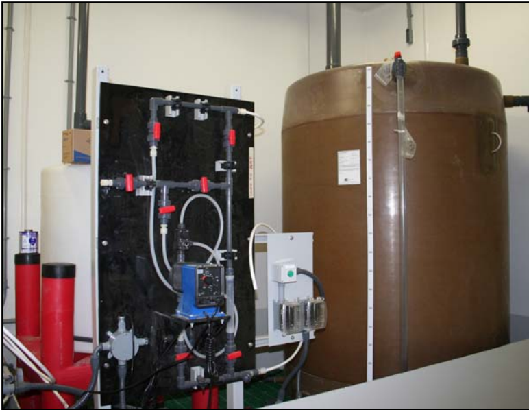
A well head Hypochlorite Feed System with bulk storage, day storage, transfer pumps, feed pumps and controls in a pre-assembled building.
