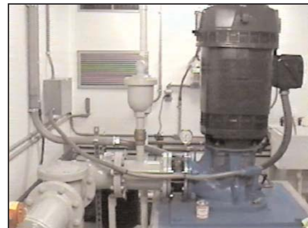
Station placed over wellhead and connected and grouted into place.
