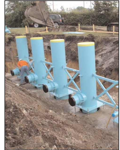
Site installation of buried pump barrels assembly.
