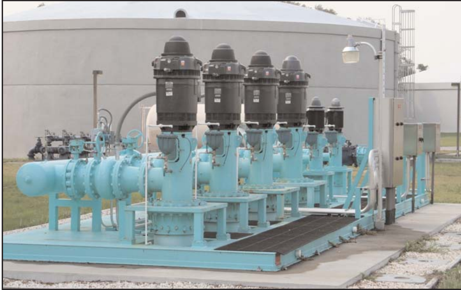
Skids dielectrically isolated from the concrete and ferrous component.
