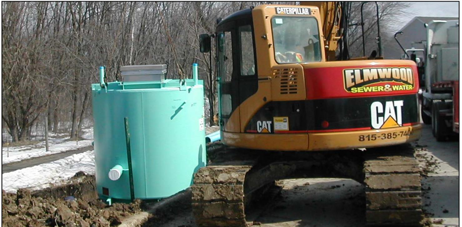
Here is one of the pressure reducing stations being set into place. After installation is complete, an EFI factory service technician will start-up the stations and train the operators.
