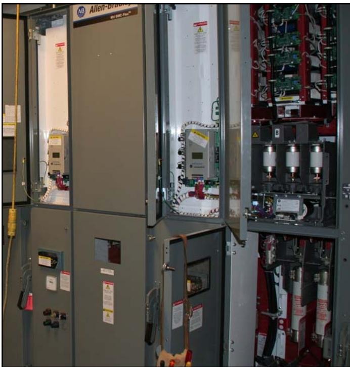
Motor Control Center (4160 Volt) being assembled. Each half of the building had its own set of pumps and controls with separate power feeds for complete redundancy.
