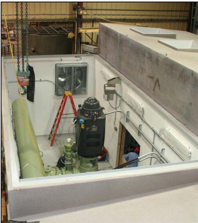
Building halves being assembled on shop floor. The buildings were assembled side-by-side at the factory, and then disassembled for shipping and final installation in the field.
