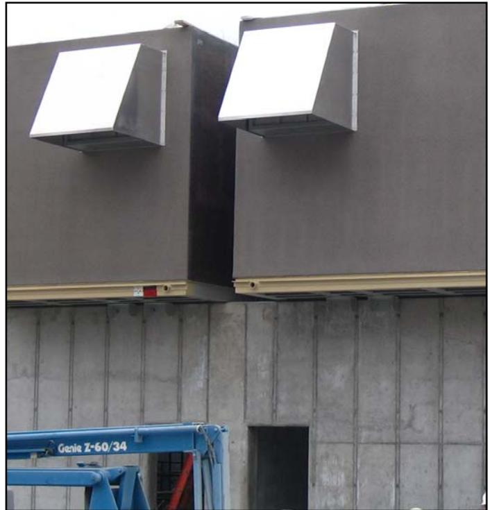
Both building halves being set into place side-by-side with the roofs to be lifted into place later.
