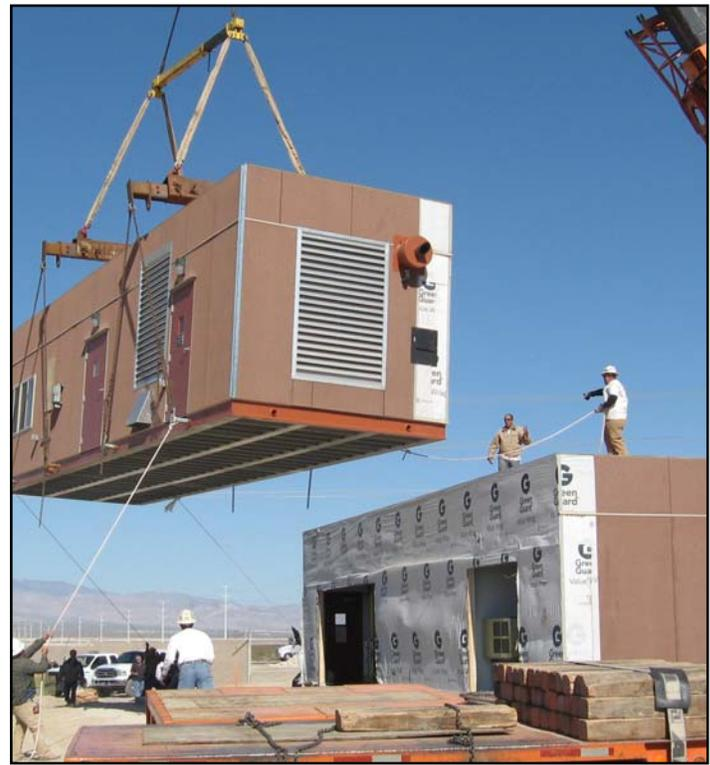
This project in Nevada is being installed side-by-side with its second half and has a desert colored ribwall exterior.
