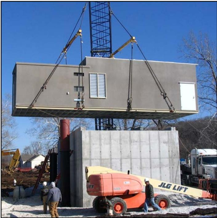
First of two building halves being lifted and placed on top of the intake structure. The low roof portion is the electrical room and is separate from the pump room.
