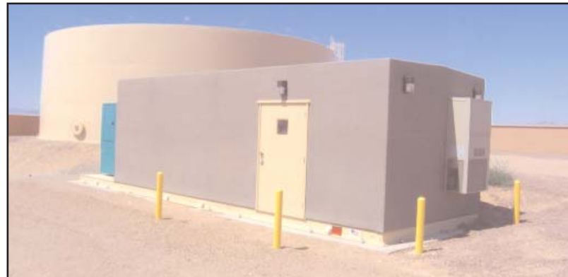
Ground service tank with pump station.
