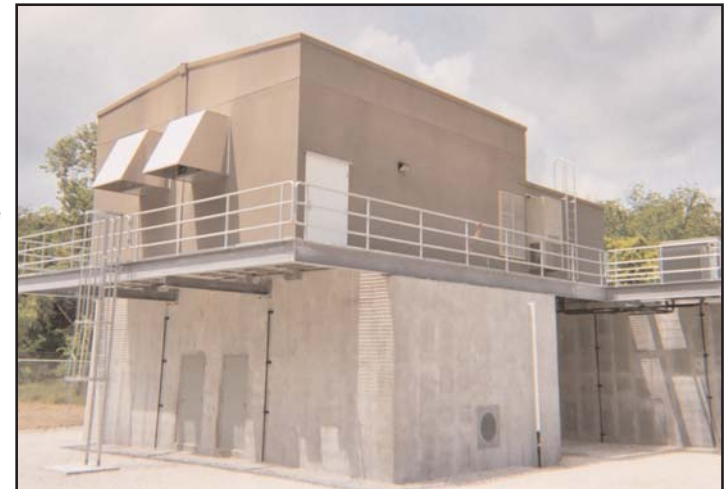
Completed Shoal Creek Raw Water Pump Station with intake structure.
