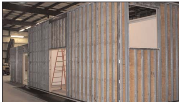
One building half in fabrication.
