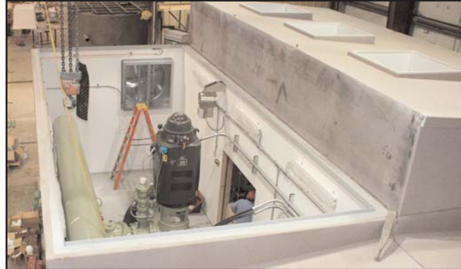
Building halves being assembled on shop floor.
