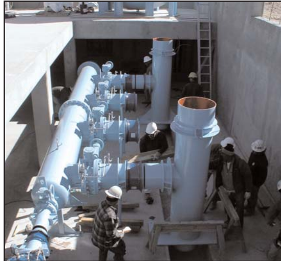
Installation of equipment.
