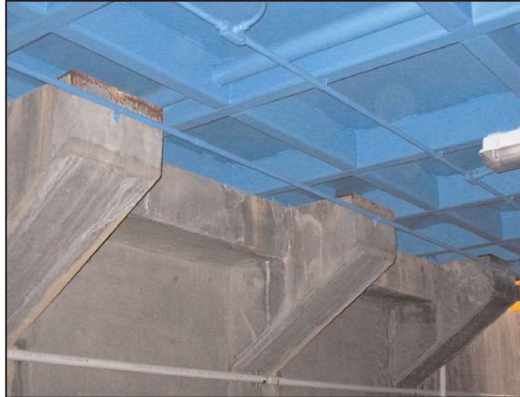
Skid support view from the basement.
