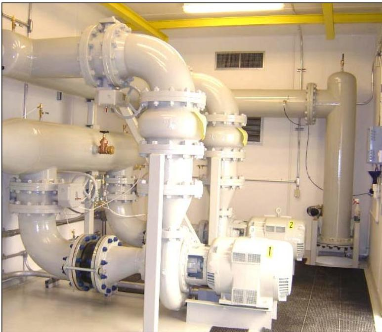
This picture shows the internal mechanical and plumbing system for the two (2) – 125 horsepower, end suction centrifugal pumps with piping, valves and support structure. The building built by EFI supports a 2000 pound capacity bridge crane for use in safely servicing pumps and valves as is required.
