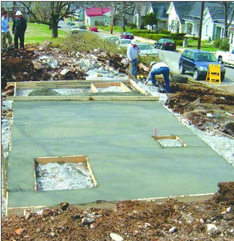
In this picture the slab-on-grade foundation is being poured. EFI provided the foundation design based on BGMU provided soil condition data.
