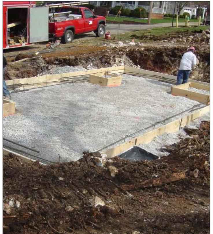
In this picture the EFI hired foundation contractor is seen forming up the simple station foundation. Disturbance of the site had to be minimal.
