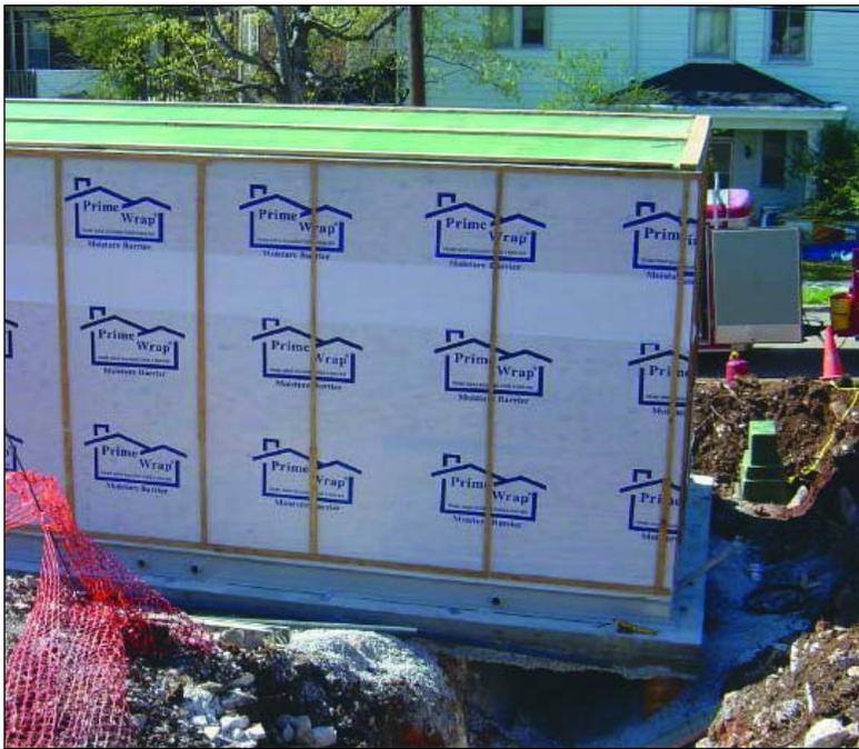
This picture shows the EFI station set in place but without the roof trusses and the exterior masonry. The truss sill boards were placed at the Factory so as to be properly anchored into the roof joist system.
