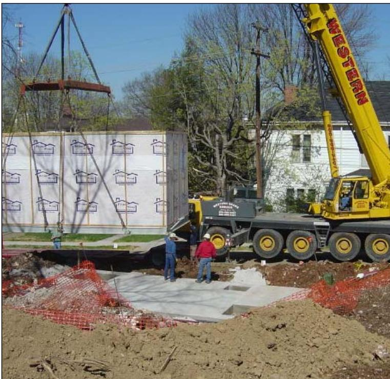
This picture shows the EFI provided crane contractor off-loading the station from the EFI delivery truck using EFI provided rigging and slings.
