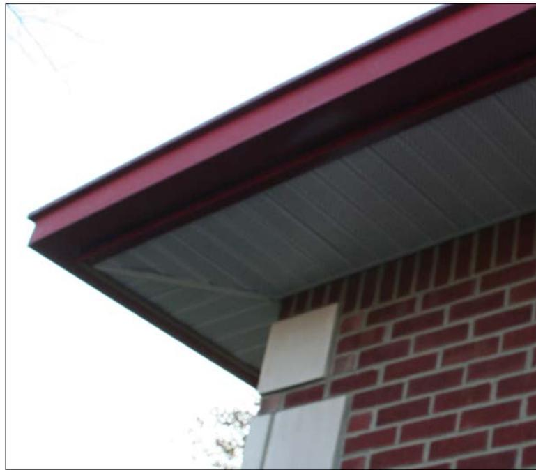
This picture shows one corner of the underside of the aluminum, standing seam metal roof, eave caps and the soffit work. The roof trusses and sheathing and the cover materials were provided and installed by a local roofing contractor as a sub-contractor to EFI.
