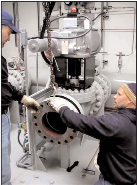
EFI pump installation crew.
