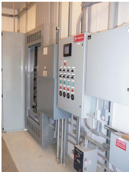
Pump controls and power distribution equipment nearing completion.
